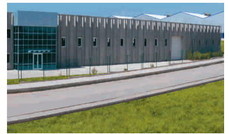
Fabrica / Factory-Eskişehir Eskişehir OSB 21.Cad. No:15 23110 Eskişehir/TURKEY Tel / Phone :+90 222 236 20 40 Faks / Fax :+90 222 236 20 49
